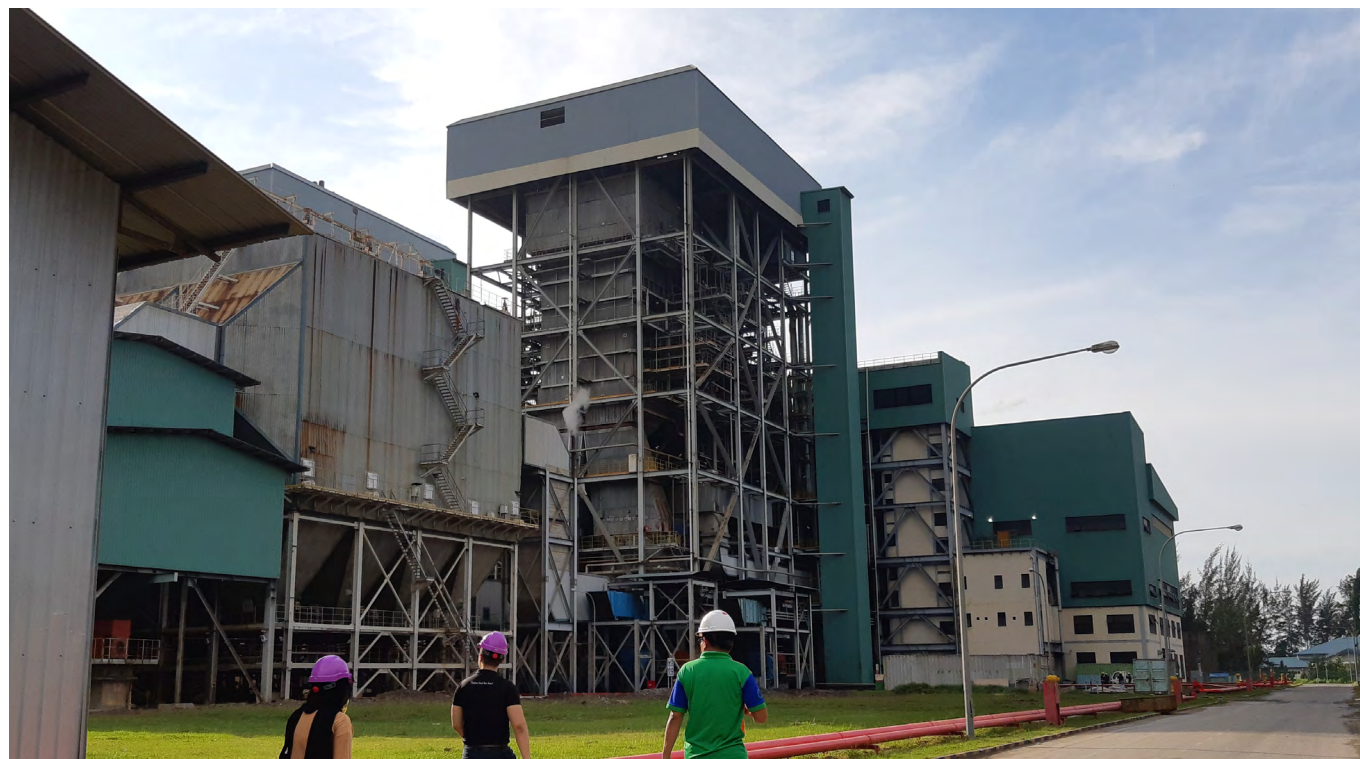
Fly ash from our coal-fired power plant is recycled as a supplementary cementitious material (SCM) in the production of cement concrete.
