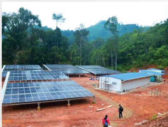
Newly completed solar hybrid system at Nanga Janan in Kapit
