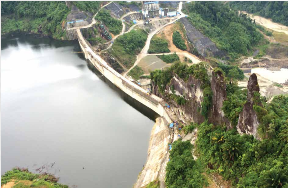
To preserve the Batu Tungun rock formation (right of picture), SEB redesigned the dam crest of Murum HEP
