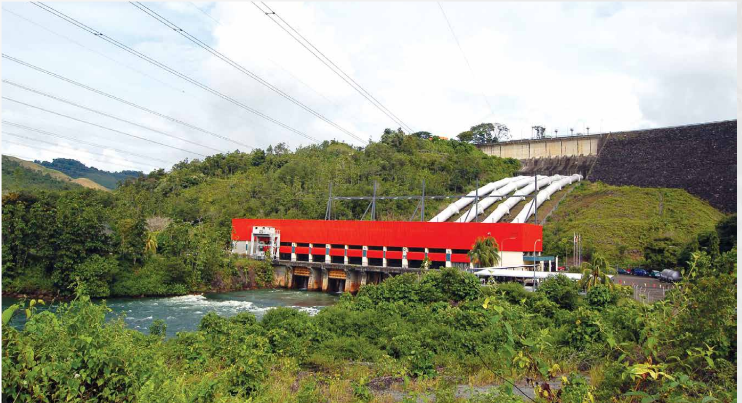
Designed to have a maximum power output of 108 MW, Batang Ai HEP was commissioned in 1985
