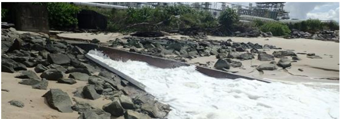
Figure 2.17 Rocks protecting the outfall located on the beach in front of power plant
