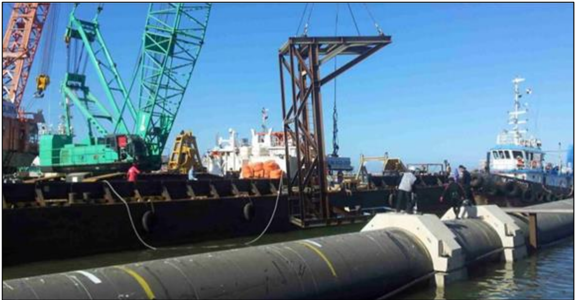
Figure 14: Example of installation of weight balancing block (source: PowerPoint for HDPE Pipeline Transportation, Storage and Assembly received on 12 th February 2018 from Sinohydro)
