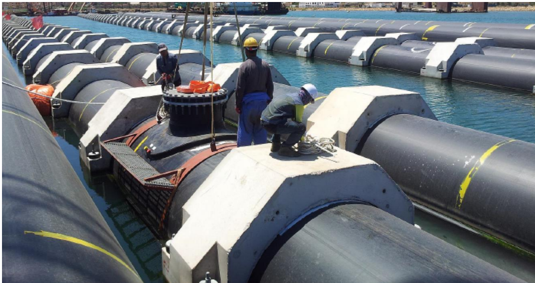
Figure 3.8 Addition of balancing weights onto the pipelines
