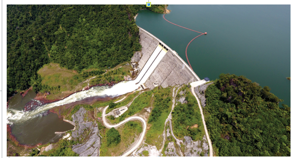
Murum Hydroelectric Plant
