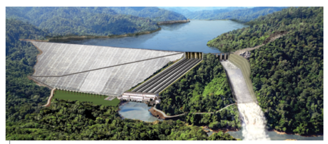
Baleh Hydroelectric Plant
