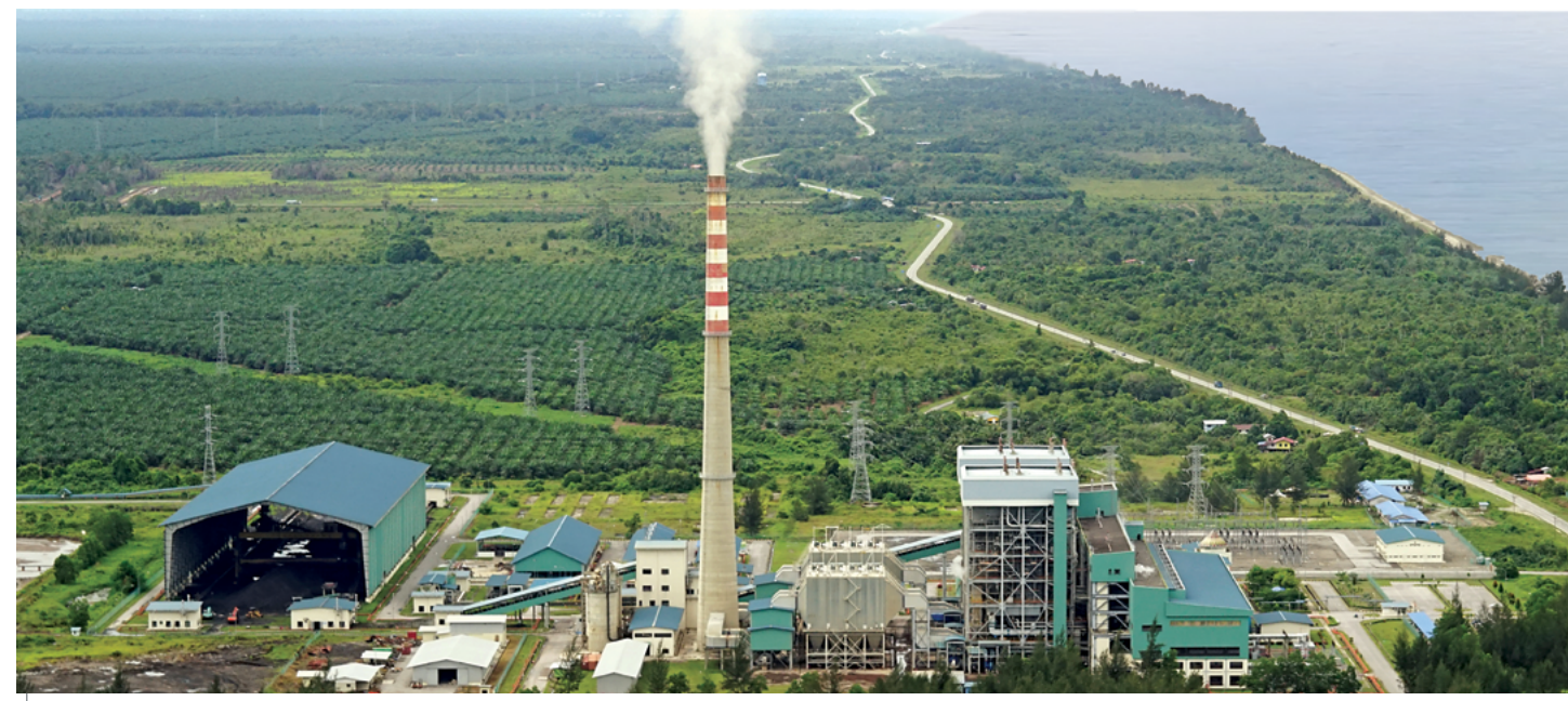
Mukah Power Generation Coal-Fired Power Plant
