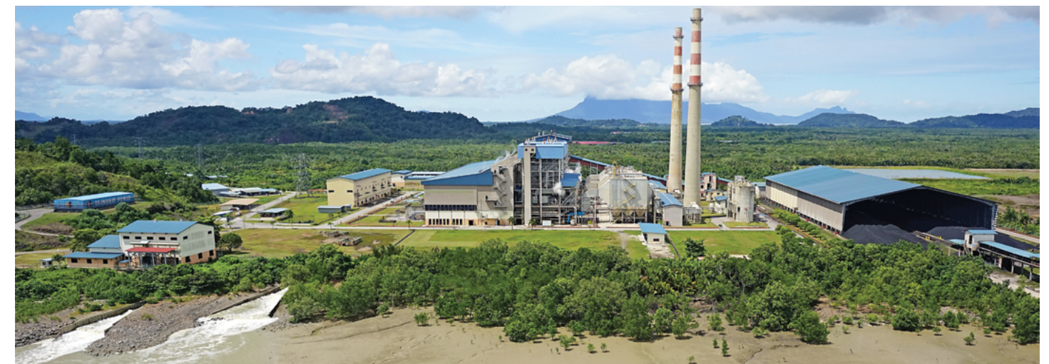
Seawater Withdrawal at Sejangkat Power Corporation Coal-Fired Power Plant
