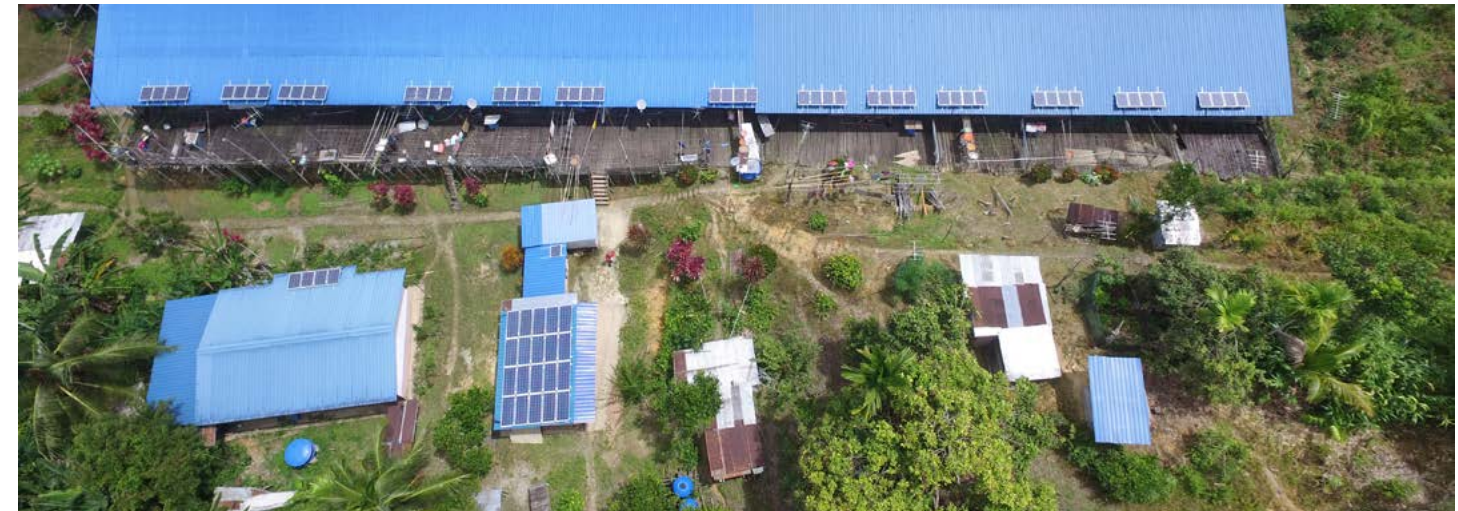
Lighting up rural households via Rural Electrification Scheme (RES), Hybrid programme, and Sarawak Alternative Rural Electrification Scheme (SARES).
