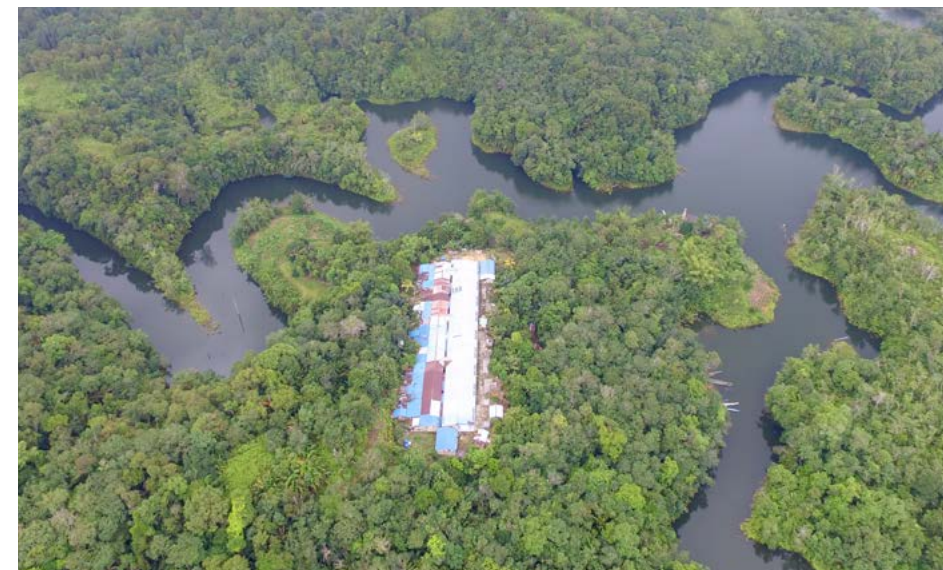
Connecting Off-Grid Households to the Grid.
