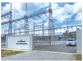
The successful and safe commissioning of the 275kV and 33kV Serudit Substations upon completion of the Engkilili-Serudit line turn-in work strengthens our current supply network by reinforcing the distribution system for Betong, Pusa, Saratok and Spaoh, and also serves as a 132kV transmission injection point into Sri Aman in the future.
