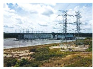
• The Samalaju B to the new Press Metal plant (PMB3) 275kV Transmission Line 1 and 2 was successfully commissioned on 11 December as part of ongoing efforts to provide reliable electricity supply to our customer. The 10km line route project is a dedicated 275kV transmission line from the existing Samalaju B 275/132/33kV GIS Substation to PMB3.
